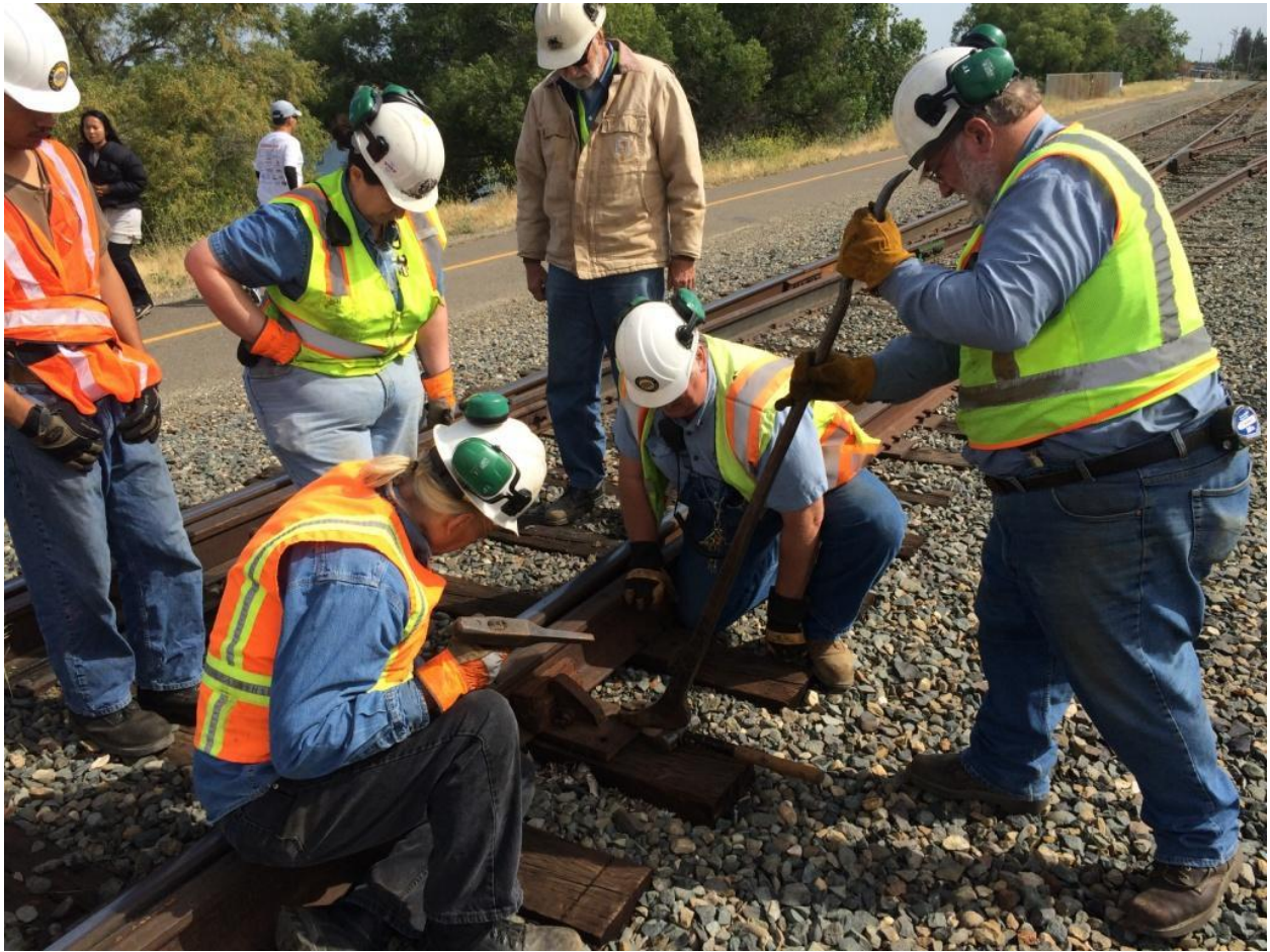
More work on Switch 13: a bracket needed a little adjustment
