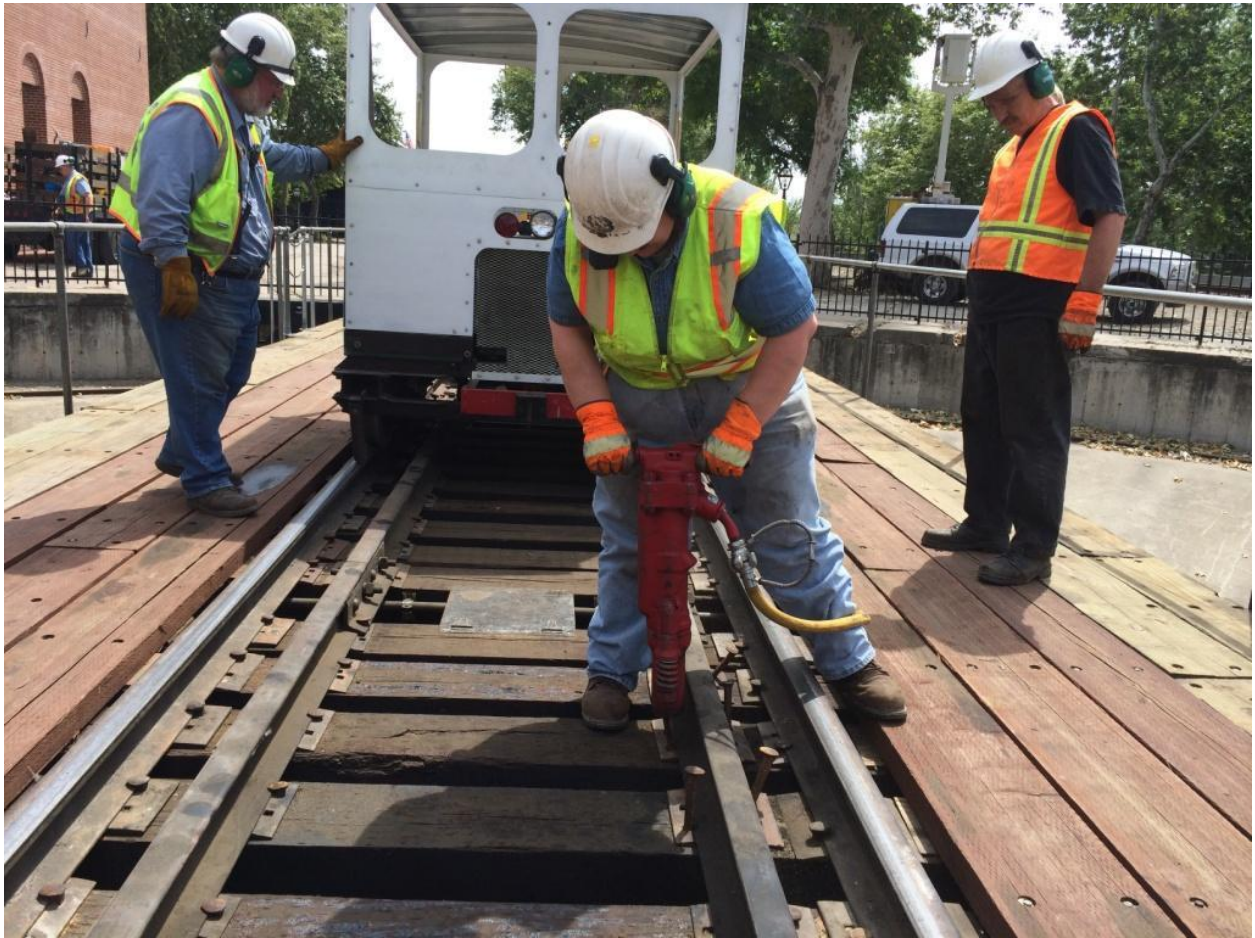
Heather fires up the pneumatic spiker and drives spikes on the turntable
