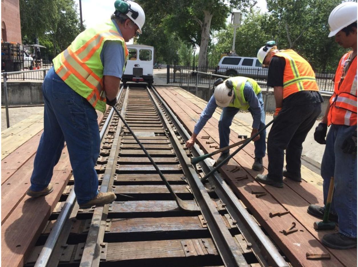
Chris nips the narrow gauge rail so that Alan and Fred can fit the tie-plates under the rail
