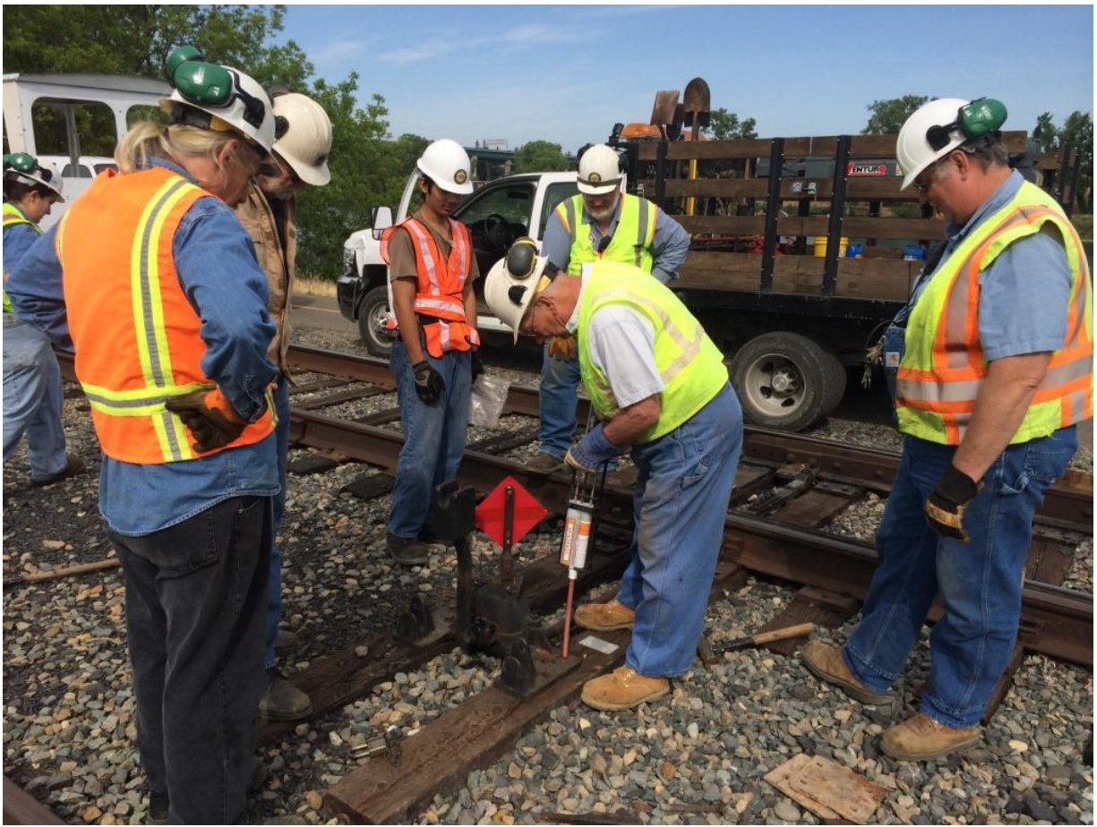
Clem injecting epoxy in the spike holes. Considering the rapt attention of Fred, Alan, Josh, Frank, and Chris, one would think doughnuts were being injected into that head-block...
